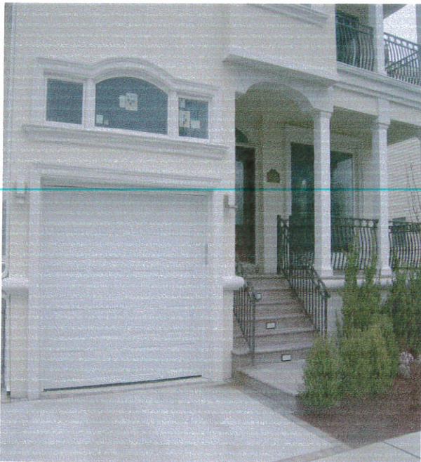
Front View Date Taken: 04/09/2008
